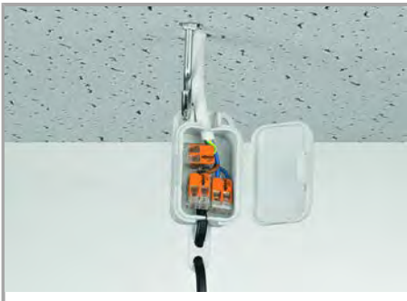
Pendant light connection in suspended ceilings
