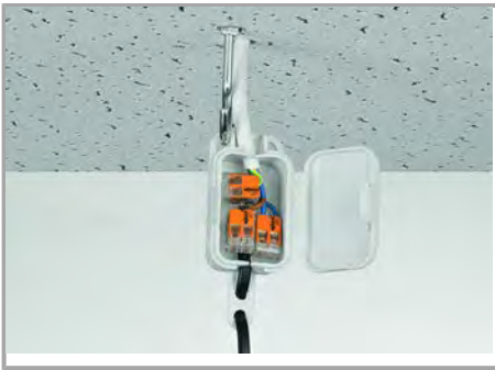
Pendant light connection in suspended ceilings
