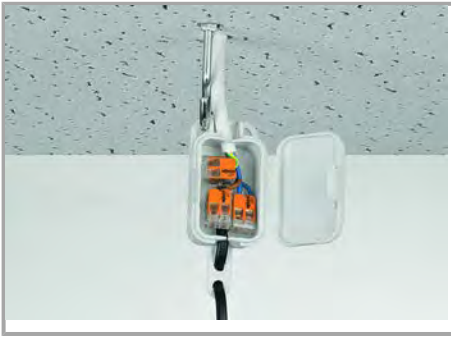
Pendant light connection in suspended ceilings
