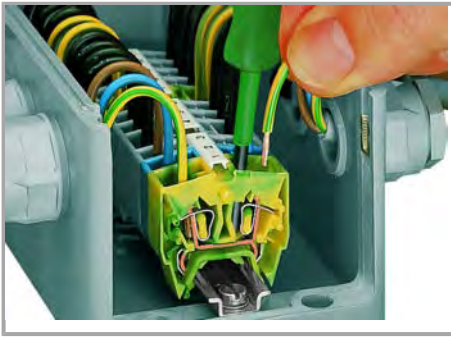
CAGE CLAMP® connection
