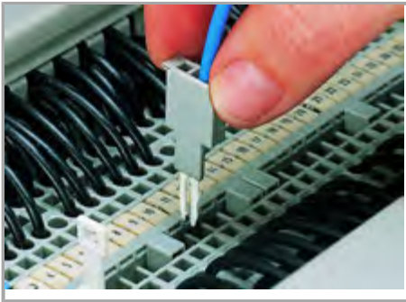
Testing with a test plug
