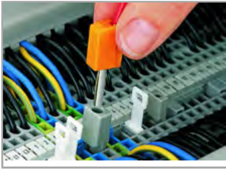
Testing with a test plug
