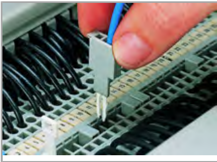
Testing with a test plug
