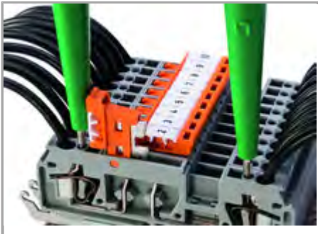
Testing with voltage tester.
