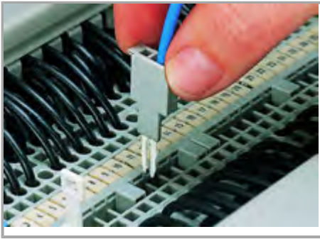
Testing with a test plug
