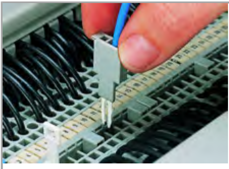
Testing with a test plug
