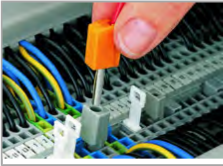
Testing with a test plug
