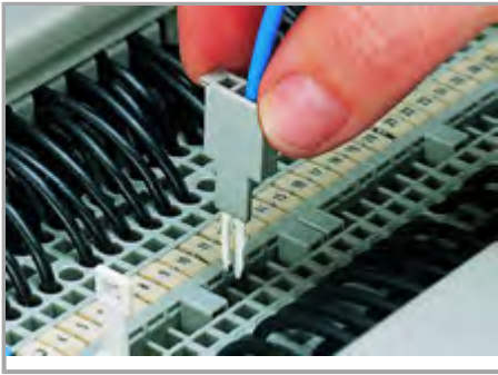
Testing with a test plug
