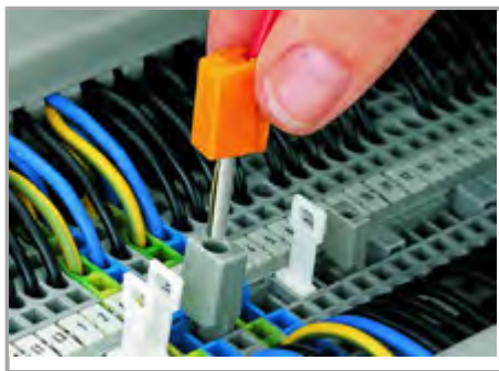
Testing with a test plug
