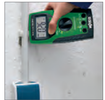
Close proximity voltage measurement
